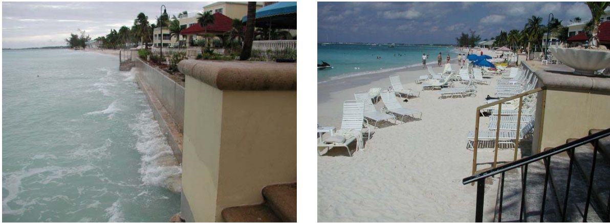
Figure 2. Before and After Breakwater Installation Photographs – View North October 2002 (left) and February 2003 (right)
