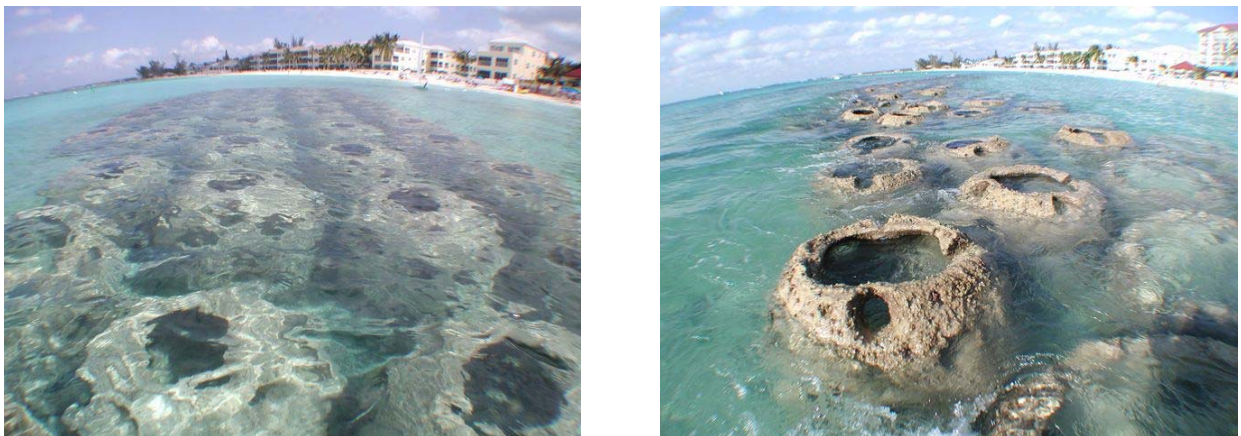
Figure 11. Northern (left) and Southern (right) Reef Ball Artificial Reef Submerged Breakwater Segments at Extreme Low Tide.
