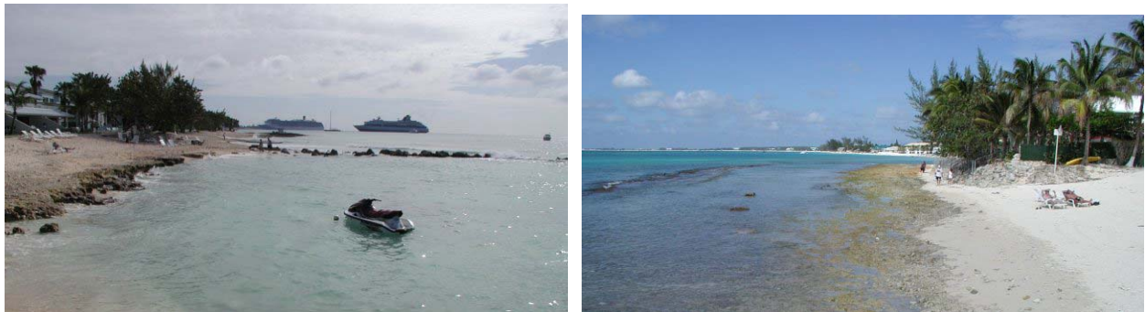
Figure 4. View SW towards the Port showing the existing Groins south of the Marriott (left); and view N towards Seven Mile Beach showing the rocky coast south of the Marriott
