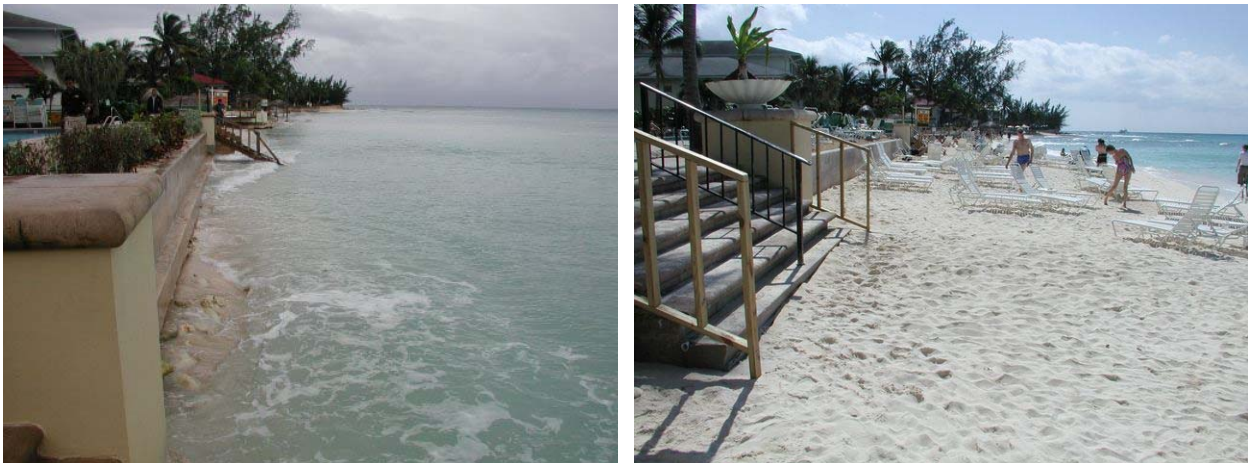
Figure 1. Before and After Breakwater Installation Photographs – View South October 2002 (left) and February 2003 (right)
