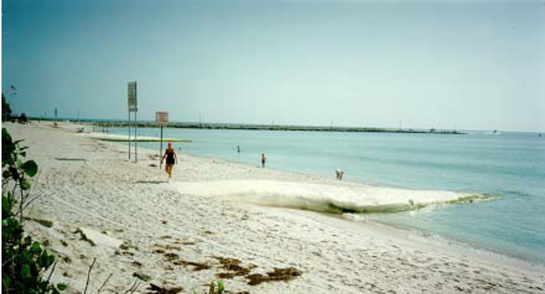
Figure 6. Sand-filled Groins Stabilizing a Florida Beach
