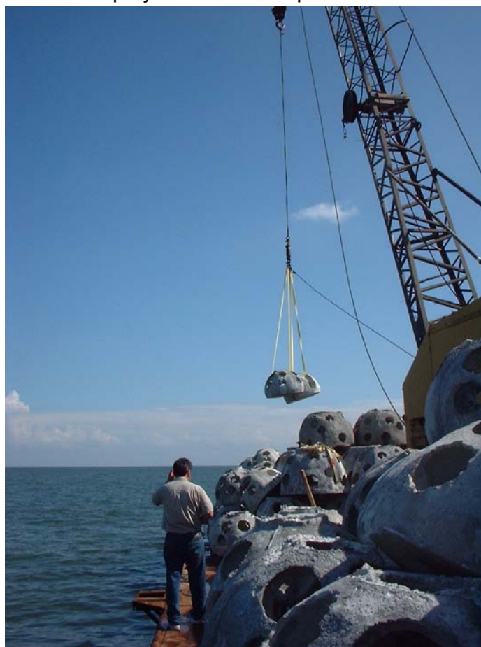
Deployment of H4 September 2003
