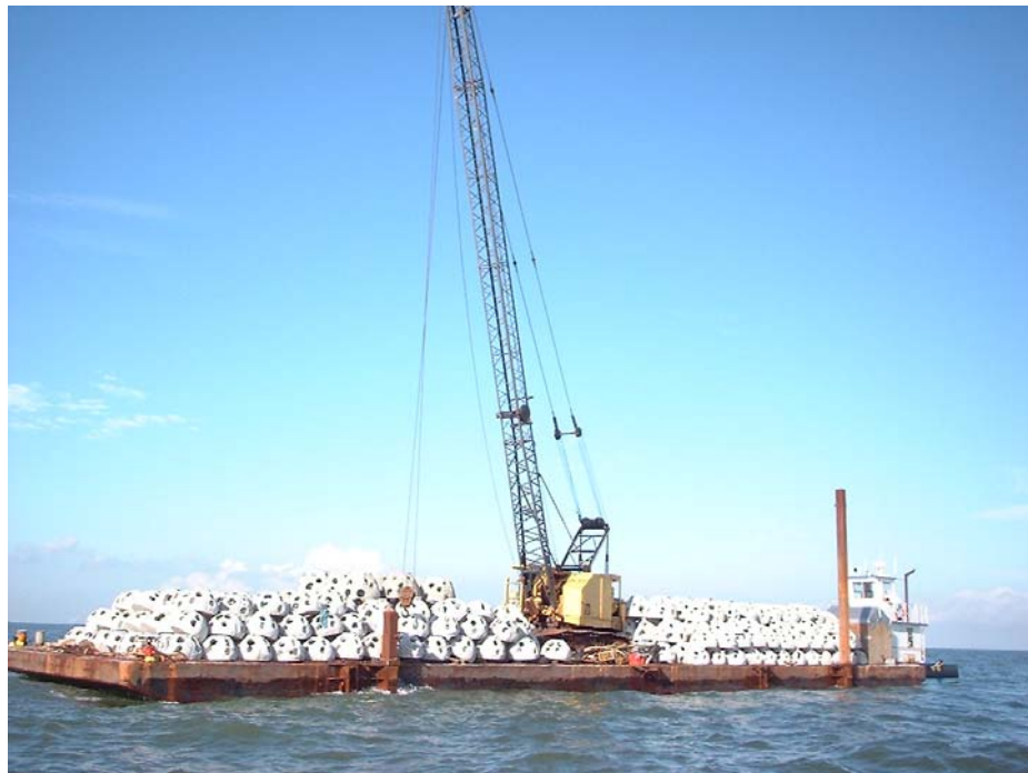
Coastal Reef Builders barge for deployment of H3 and H4 September 2003.
