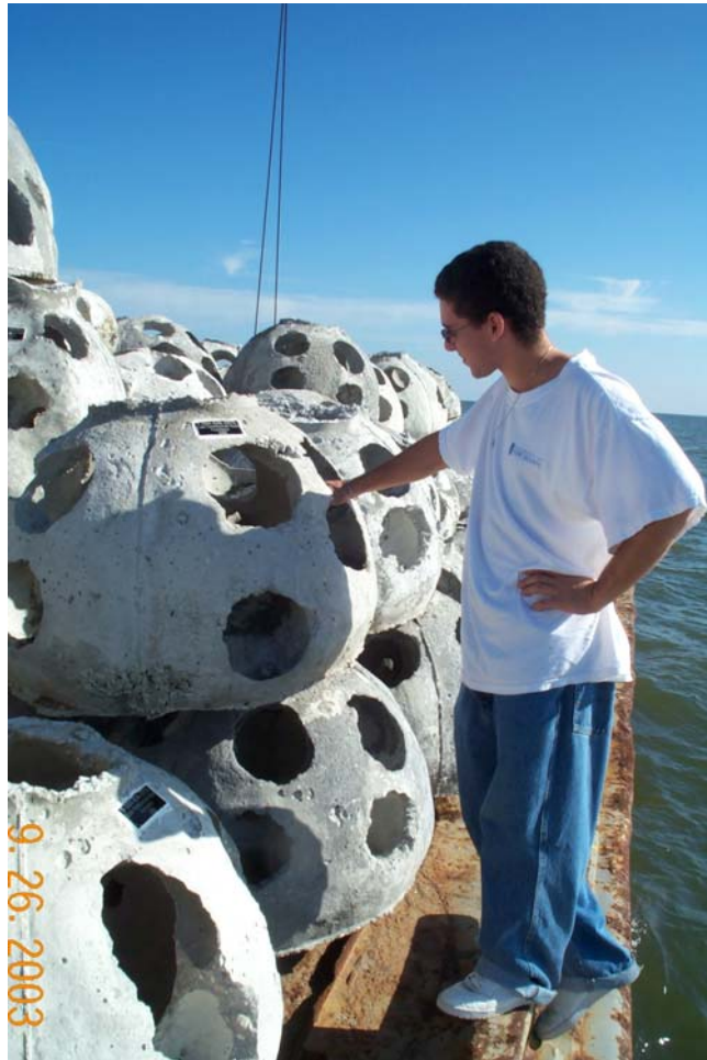
Close-up's of stacked reef balls on Coastal Reef Builder's barge.
