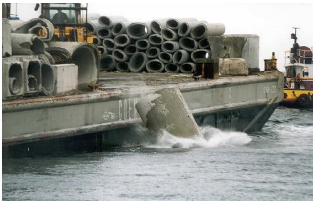
Approximately 1,100 tons of concrete castings, pipes and culverts were deployed in July 2006 to construct a "drift fishing" area on the reef site. 700 concrete reef balls were also placed on the reef.
