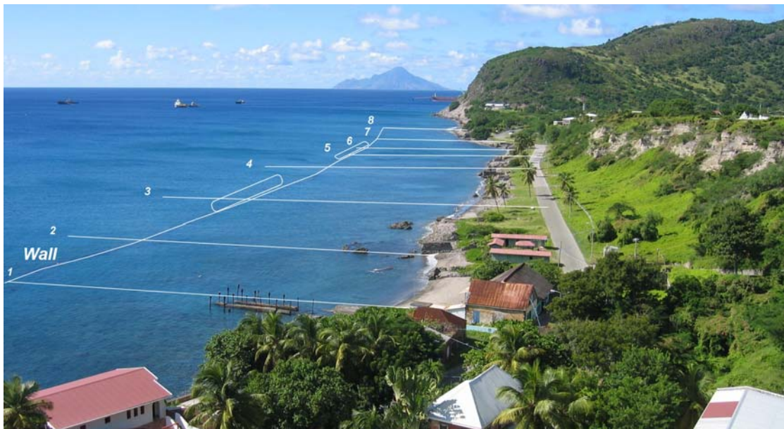
Figure 23. View North showing the Locations of the Center and Northern Breakwaters.
