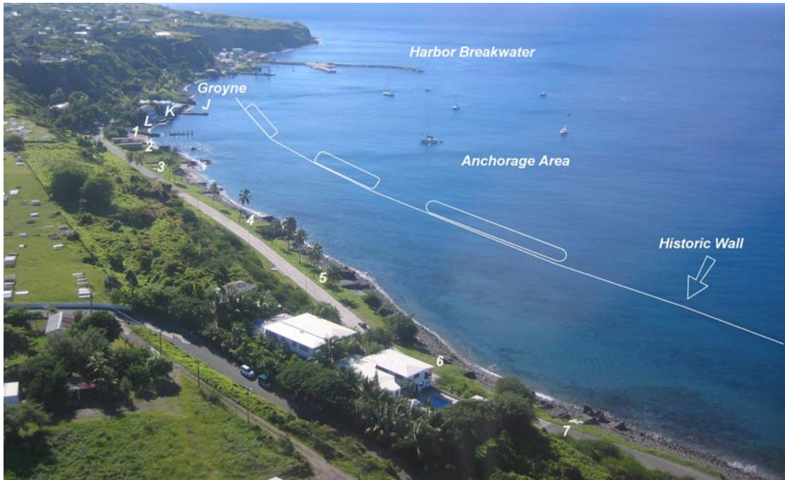
Figure 22. Aerial View of the Locations for the 3 Submerged Breakwaters.
