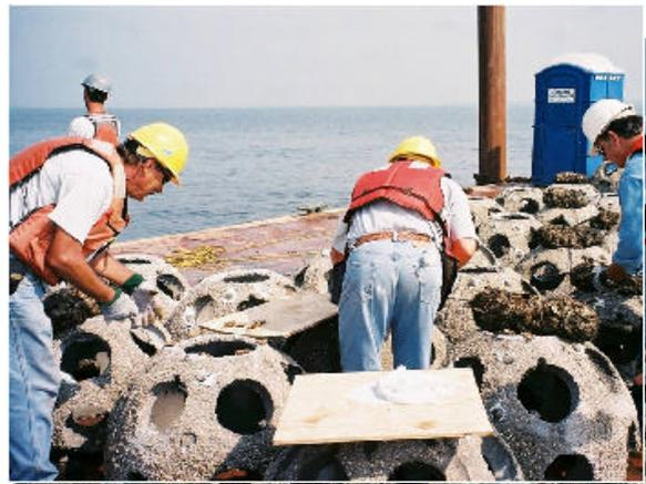
Figure 0 Maryland Environmental Service volunteers attaching plugs with oyster spat to Bay Balls just prior to placement on Memorial Reef. Photo: Wayne
