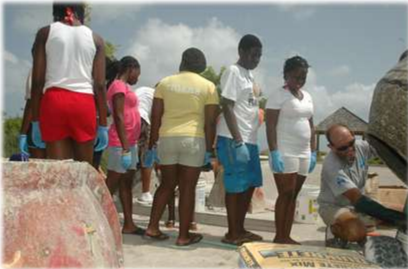
Queing up to get the buckets of concrete.
